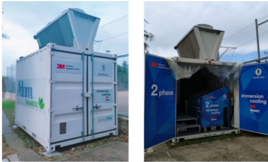
FIGURE 8 Two-phase immersion cooling EDC prototype.
